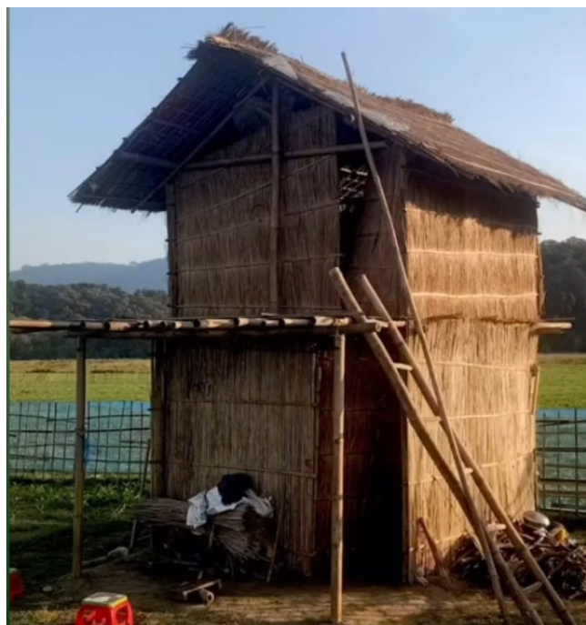
Figure 1: Traditional Chang Ghar built with bamboo and hay straws
