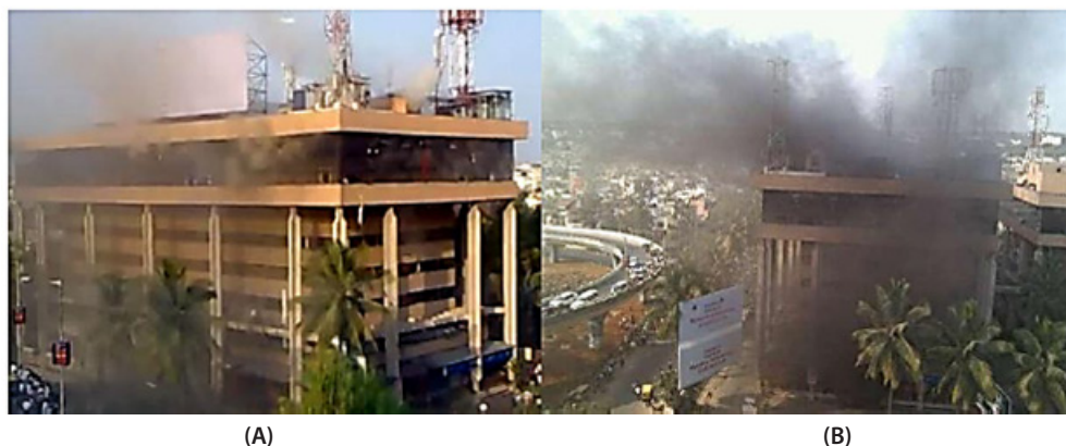
Figure 7: (A) Carlton tower-Under fire; (B) Carlton tower-the extent of smoke
