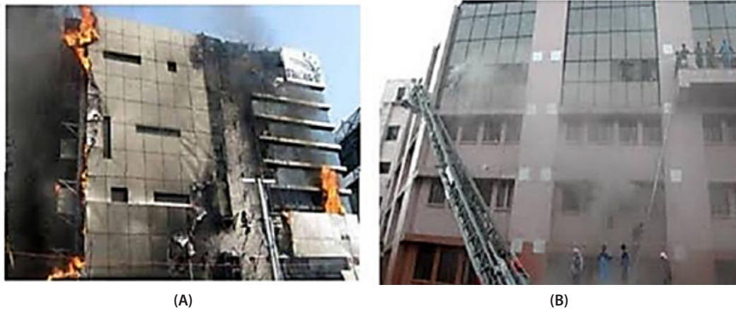
Figure 6: (A) AMRI Hospital- -under fire; (B) AMRI Hospital- -Glazed Facade
